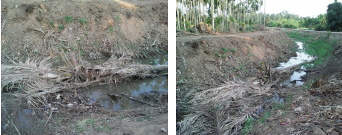
Plate 5: Vegetation clearance for site access in Sanyasikodmagge area of Gondhi System
