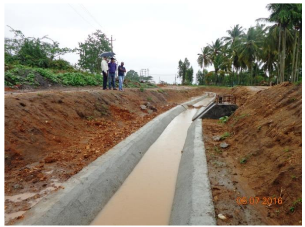
Canal lining work in LBC tail end
