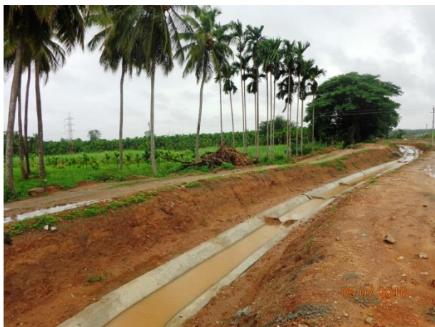
Canal lining work in LBC tail end
