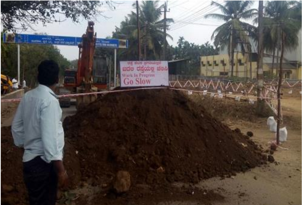
Safety Signboards at Construction Site
