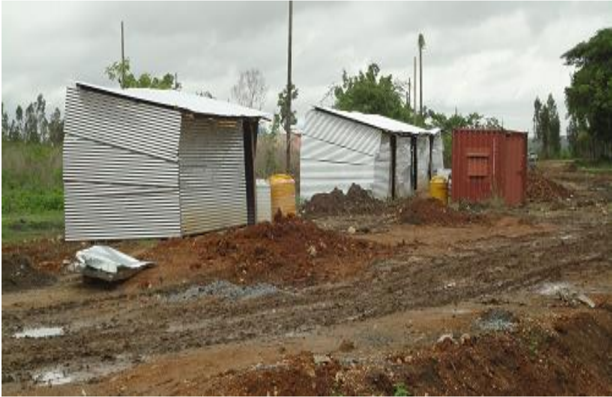
Make-shift Labour Quarters provided by the Contractor with Water and Sanitation Facilities
