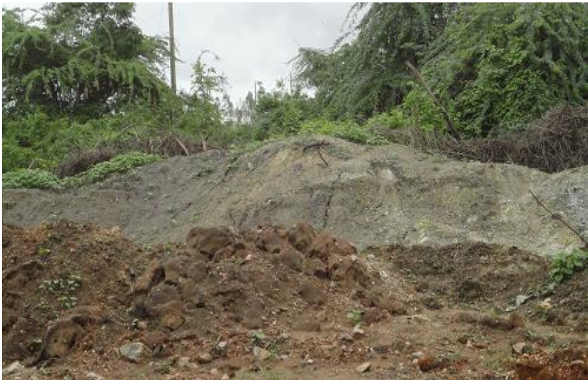
Disposal of Silt as initially practised by the Contractor-June 28, 2016
