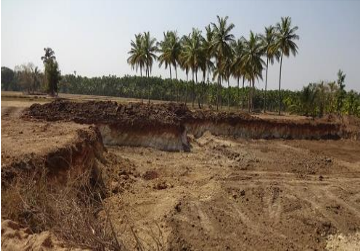
Burrow Site used for Right Bank Canal Rehabilitation Work
