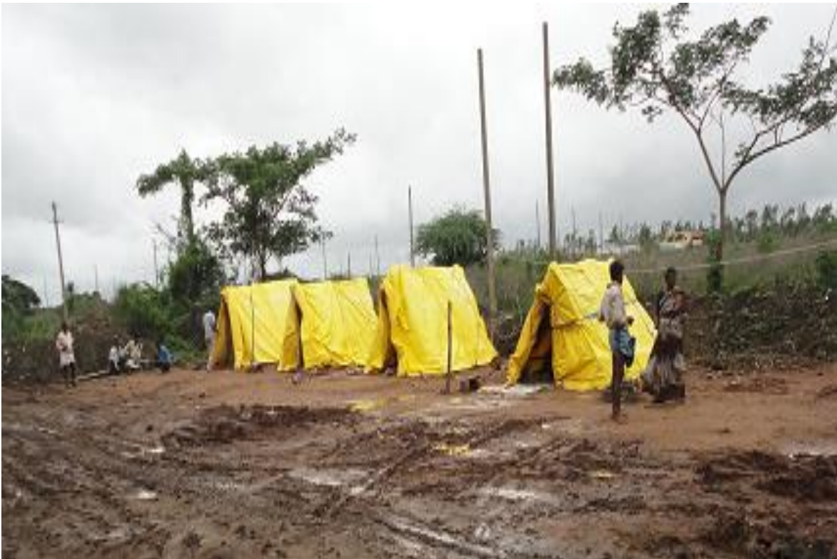
Temporary Shelters provided by the Contractor for labour for short breaks–June 28, 2016
