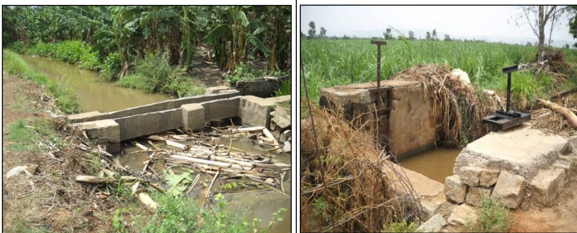
Fig 13.3 – Channel used as disposal point
