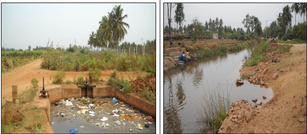
Fig 13.2 – Figure showing untidy channels
