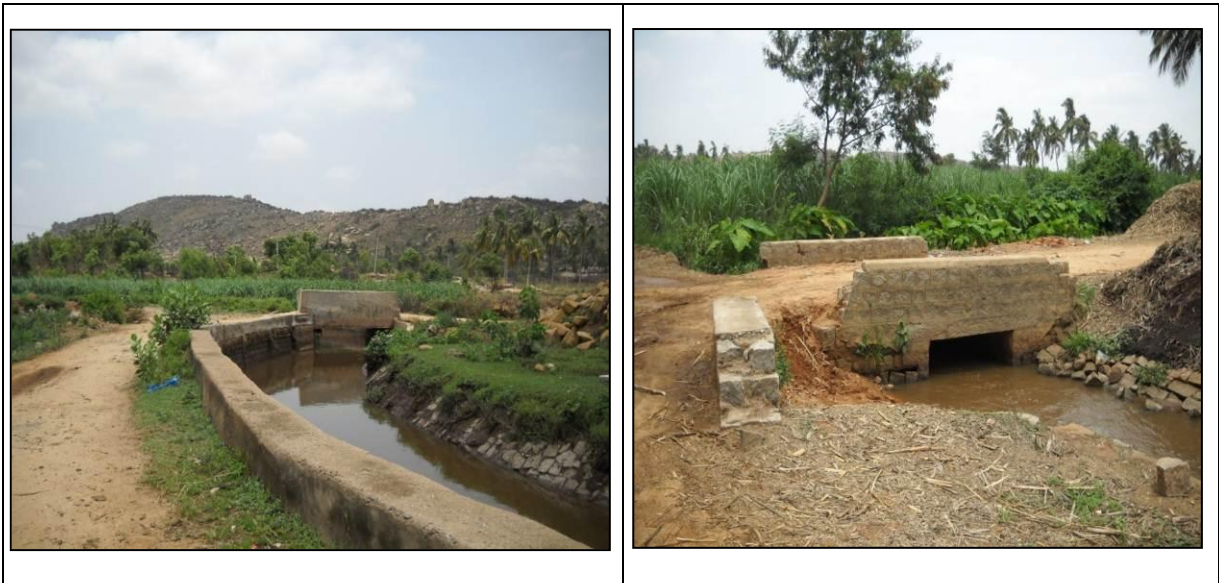
Fig 13.4 – Channel reaches with size stone masonry lining
